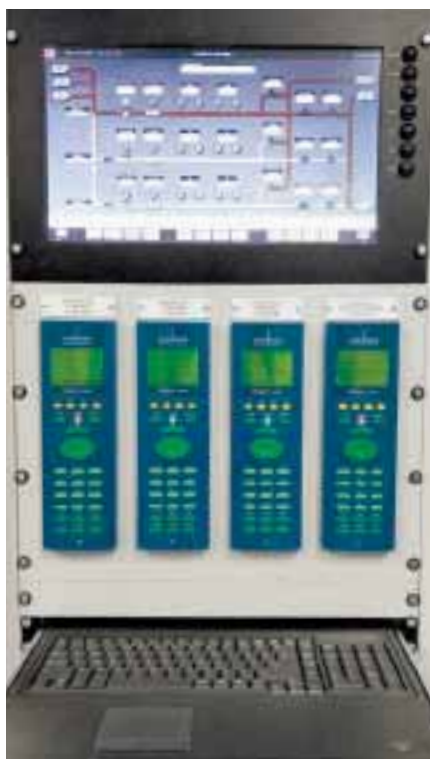
A control panel with a metering supervisory computer and Emerson S600+ flowcomputers
